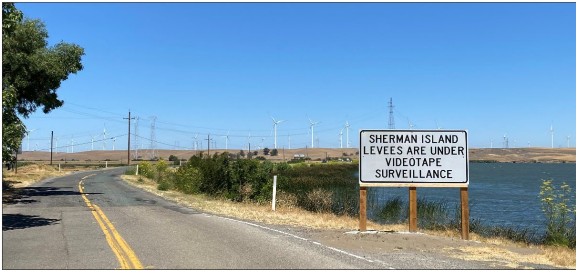
Figure 10. Security Camera and Signs
