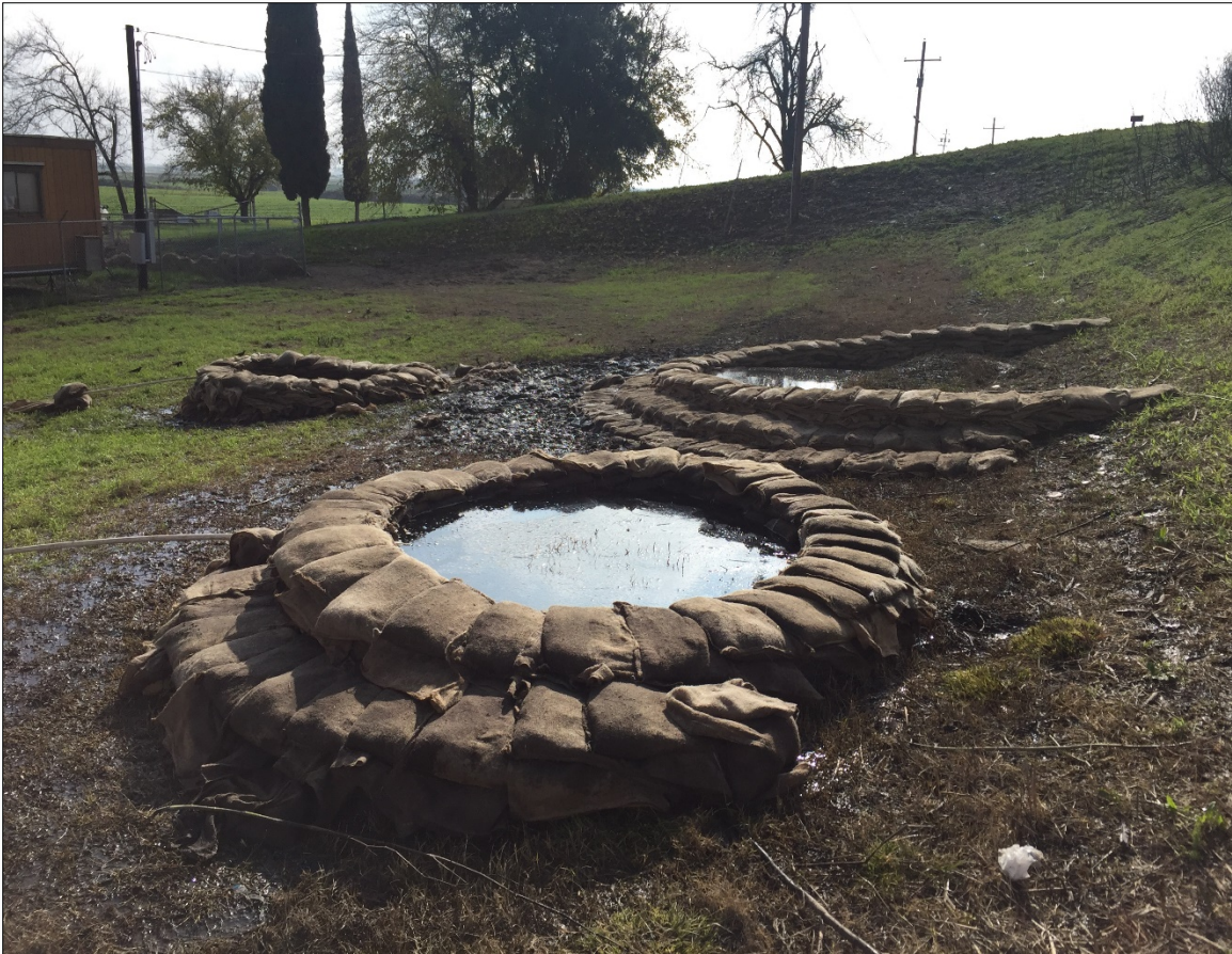
Figure 5. Boils at Sta. 960+00
