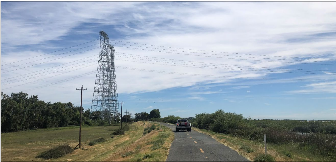
Figure 12. Transmission Lines at Sta. 300+00
